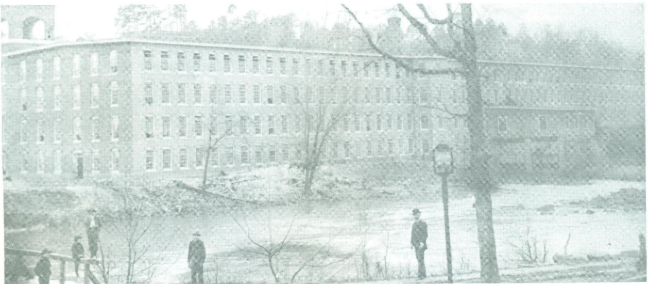
Pacolet Mill 1 & 2 destroyed in 1903 by flood.
