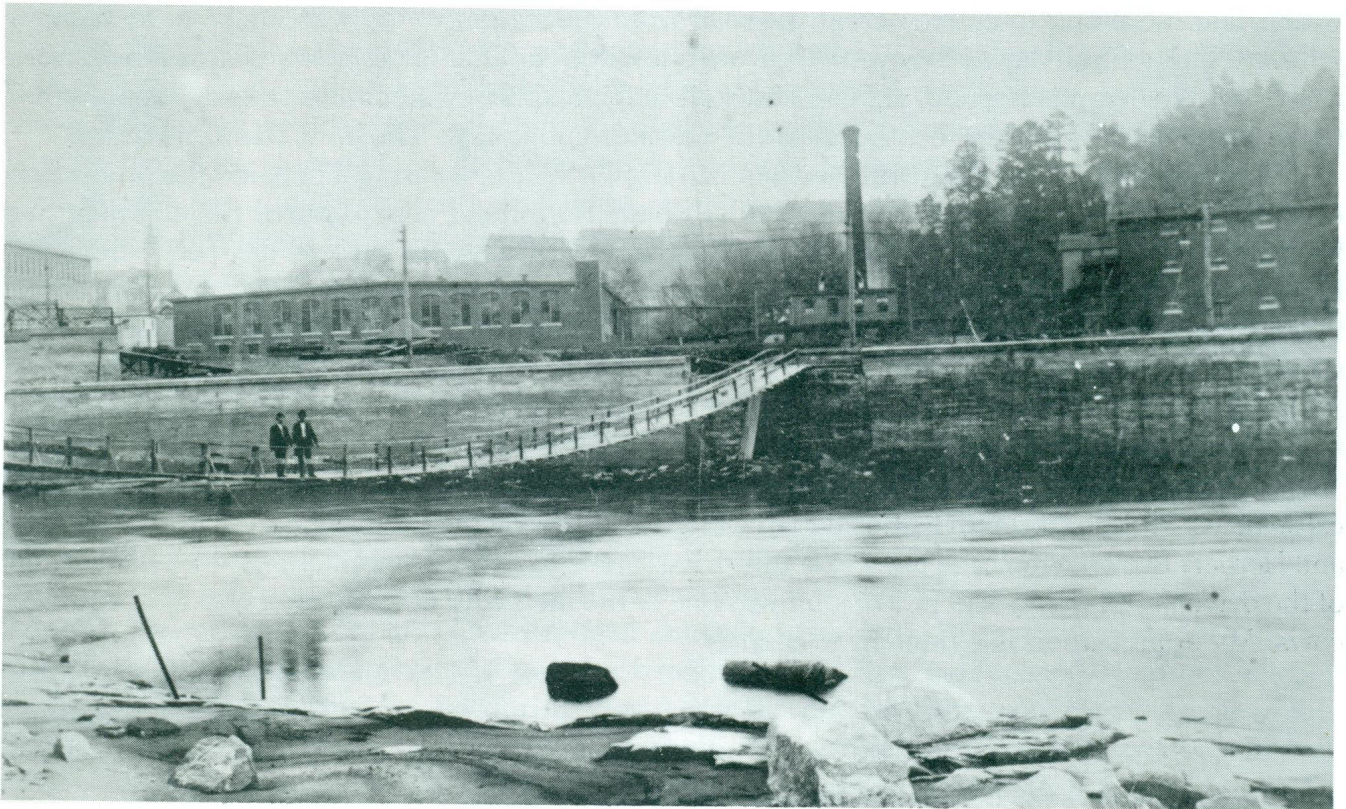
This temporary swinging bridge was used while a steel constructed bridge was being built to replace the bridge that was destroyed by the high waters of the Pacolet River in 1908.
