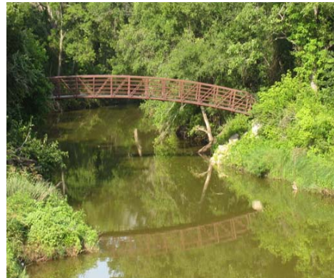
Figure 4.3 Example of a Pedestrian Bridge
