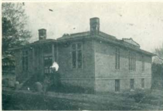
THIS METHODIST CHURCH WAS REPLACED ABOUT 1920.
