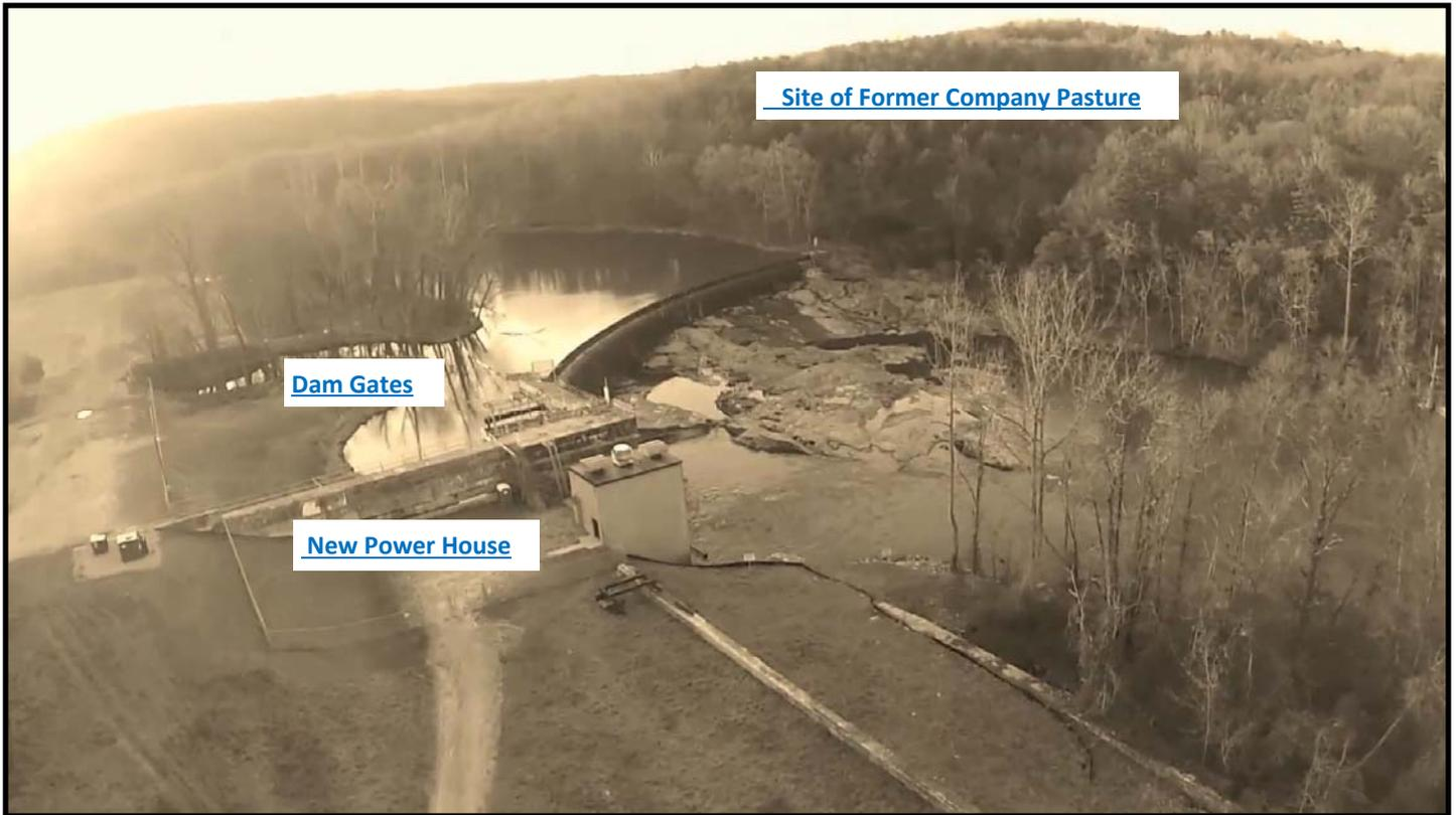
Taken from above the site of the former “New Mill” (Mill no. 5) looking up the Pacolet River toward the dam. In this view, the dam gates are drawn and the water is bypassing the dam. The rocks that make up Trough Shoals are exposed. The old Company Pasture was across the River. The new power house was recently installed by The Lockhart Power Company. It uses water power from the dam to generate electricity for its customers.
