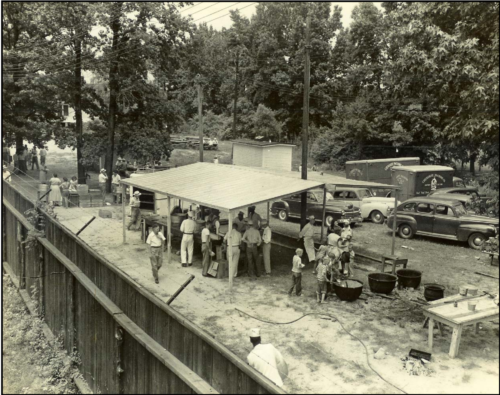
Area where the food was cooked. This is just outside the ballpark on the first base side. The pit in the ground where the hogs were cooked can be seen in the right center of the picture. The large cast iron pots are where the hash was cooked.
