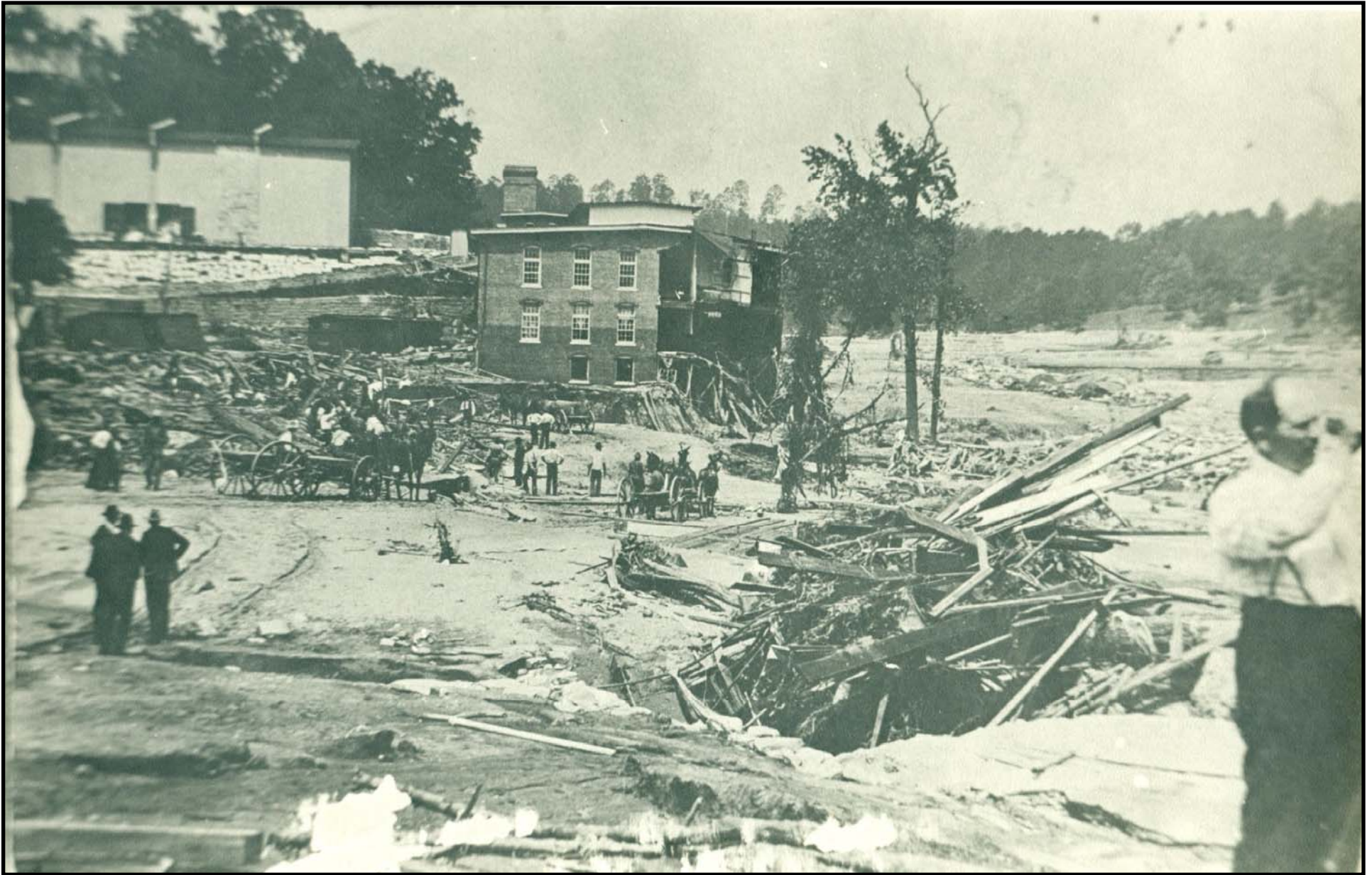
A photo of the Flat area after the Flood . This photograph was taken at ground level generally from in front of where the Girl's Club was once located.
