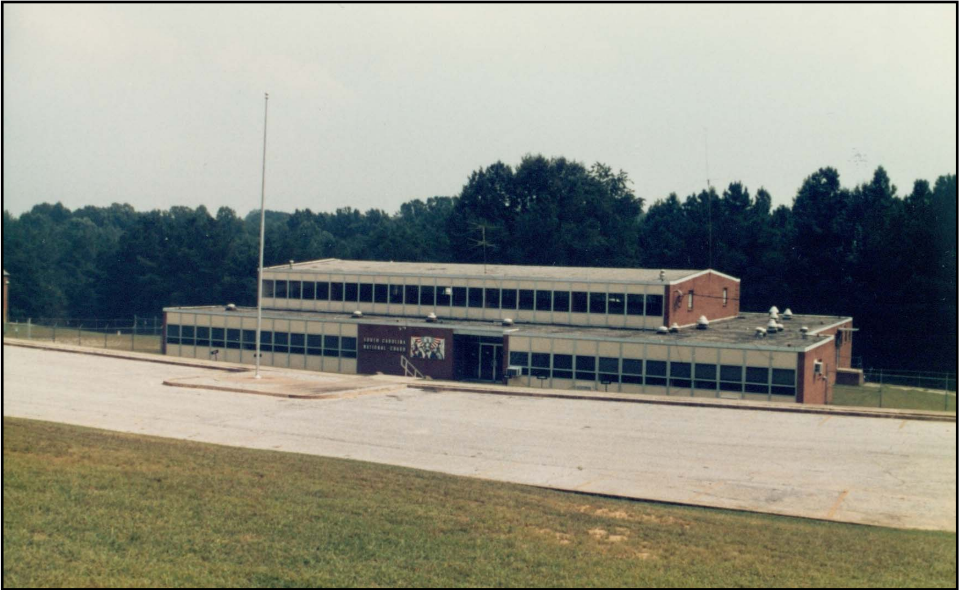
The National Guard Armory on Sunny Acres Road. It was built in the early 1950's and is no longer used. For many years it was the home of the Pacolet National Guard Unit. In the 1950's the unit had several tanks and these could sometimes be seen driving on the roads near the armory.
