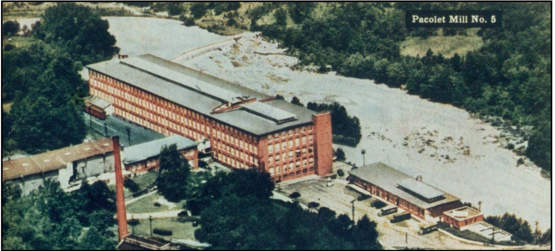
This aerial photo of the New Mill appeared in an advertisement of the Saco - Lowell Company in 1949.
