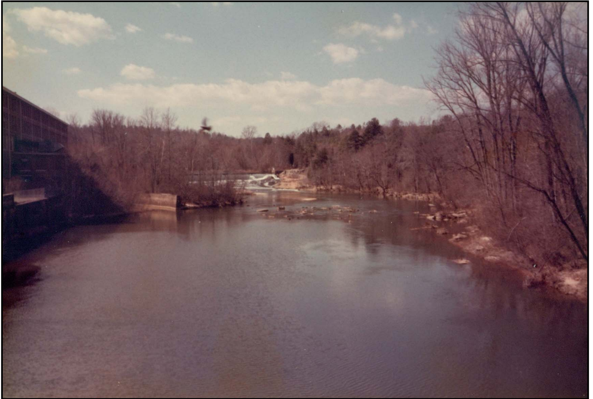
This view looks up the Pacolet River toward the dam . The New Mill (No. 5) is still standing as seen in the left side of the photo. A view of the same scene today is shown on page 6.
