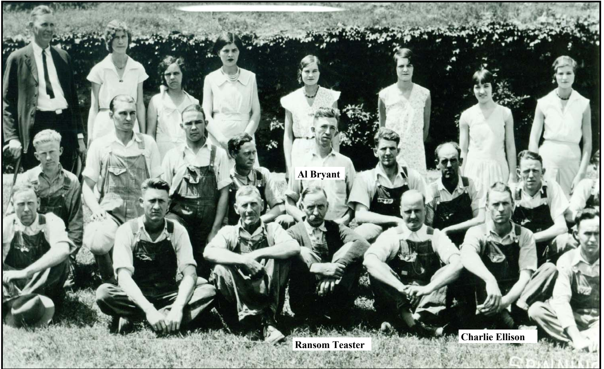
The left side of the panoramic photo for the Spinning Department of the “New Mill”, Mill No. 5 . This picture has my paternal grandfather, Ransom Teaster. Someone in the past has made an effort to identify these folks by marking up the picture. The picture with their handwritten notes is shown on the next page.
