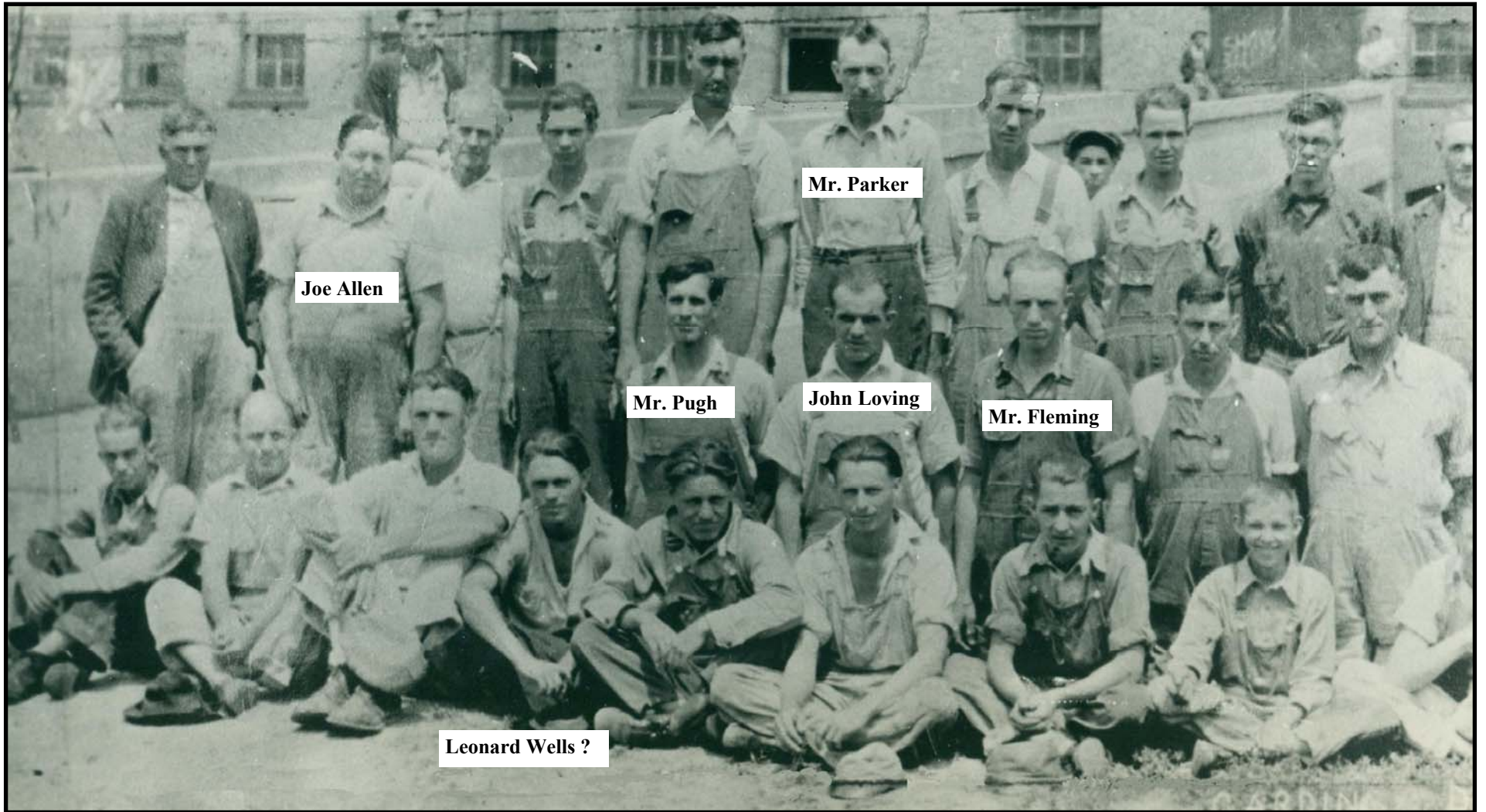
Another picture in the Oliver Photo Company series in 1931. This is a picture of the left side of the panoramic photo for the Card Room of the “Old Mill”, Mill No. 3.
