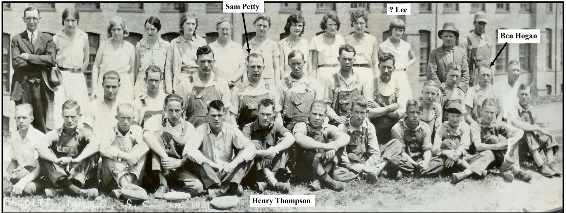
This photo is the right side of the picture shown on the previous page of the Weaving Department of the “Old Mill”, Mill No. 3.
