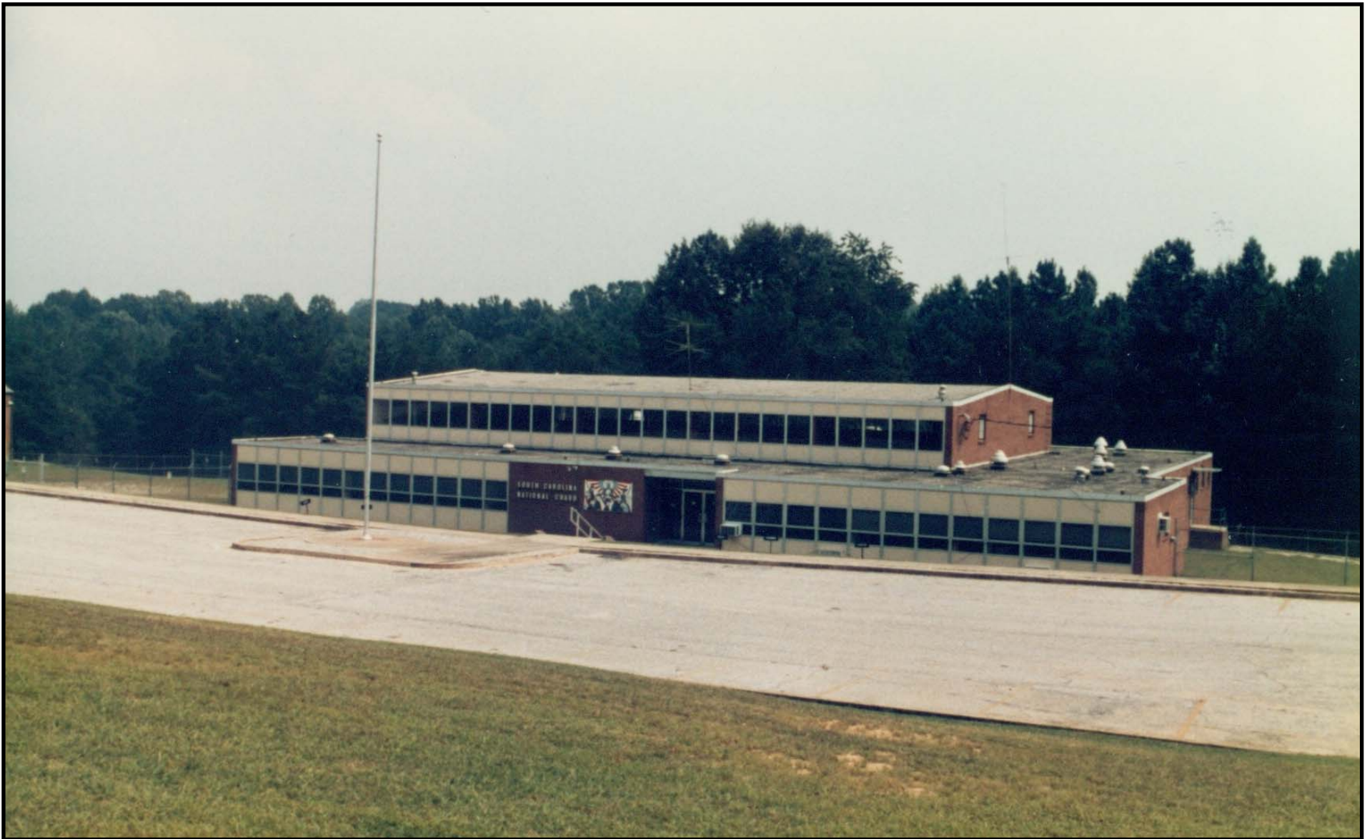
The National Guard Armory on Sunny Acres Road. It was built in the early 1950's and is no longer used. For many years it was the home of the Pacolet Mills National Guard Unit.
