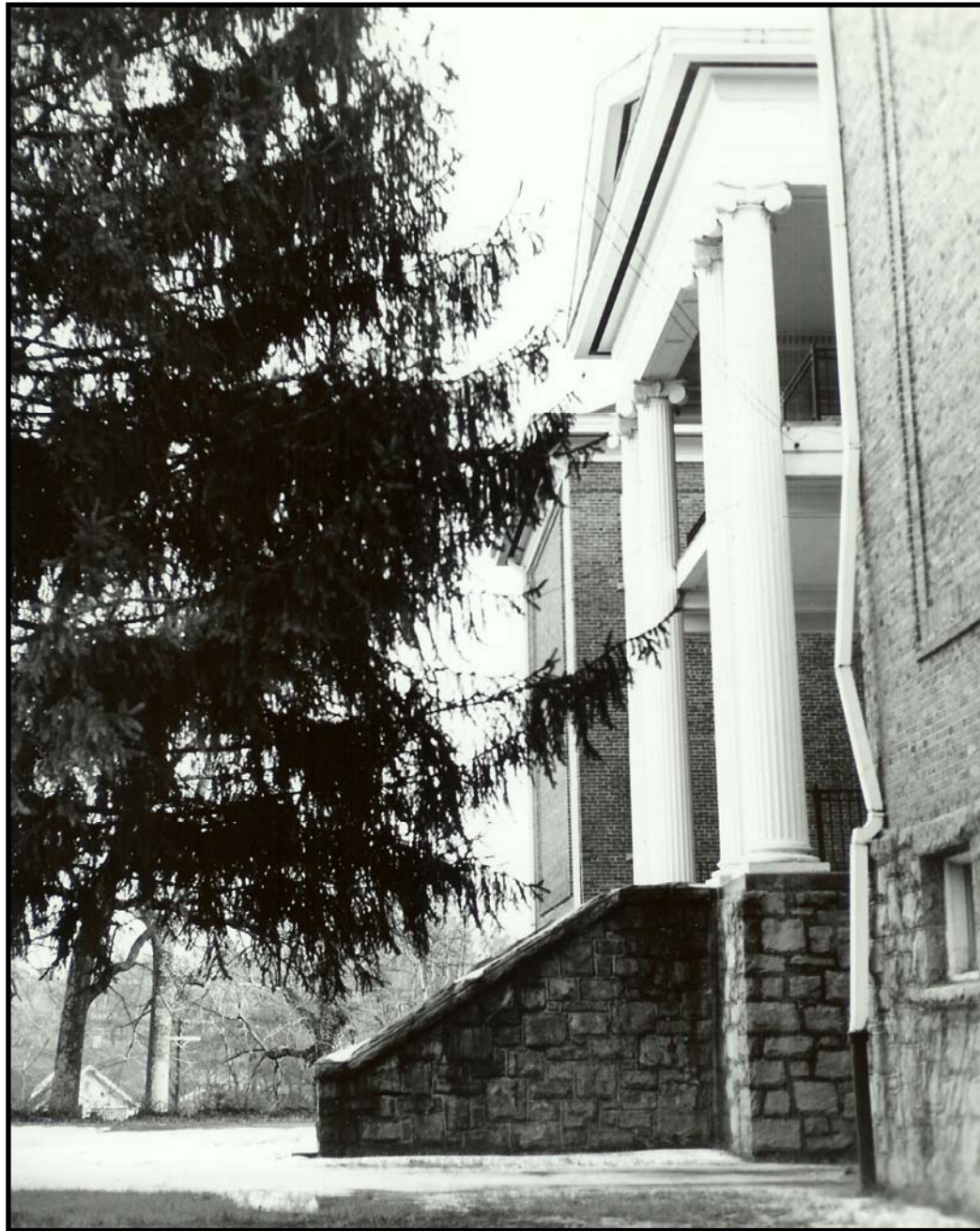
Side view of the front entrance. The Hotel can be seen in the distance.
