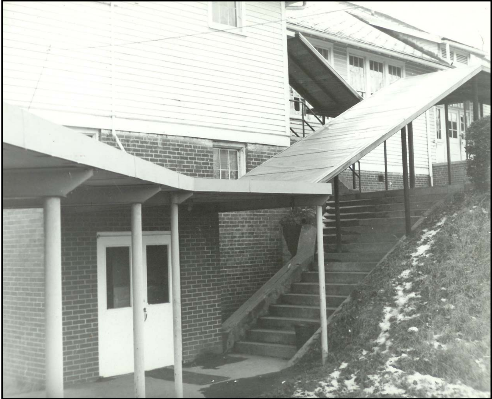
View of covered steps leading from front of Annex down to the cafeteria.
