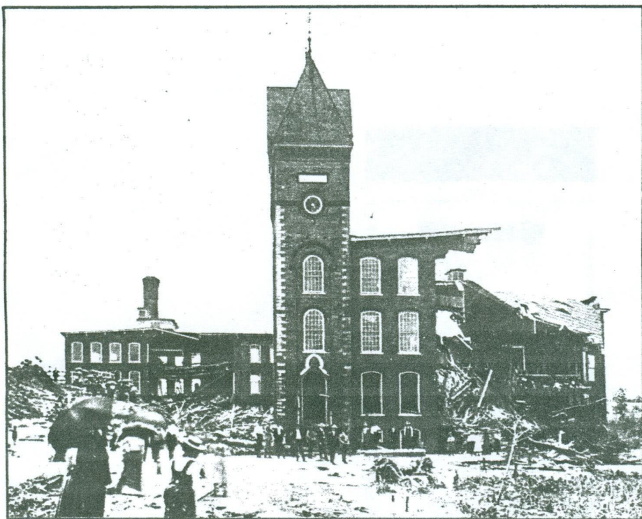
Clifton Mill No. 2 after the flood; there were 65 people killed or missing, 600 left homeless and 4,000 left without jobs.
