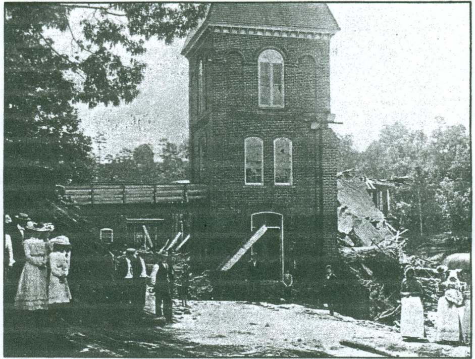
Clifton Mill No. 1 after the flood. Three persons who fled to the top of the mill were swept into the river when the roof fell in (at right). Sightseers in their Sunday best were caught by photographer June Carr of Gaffney.
