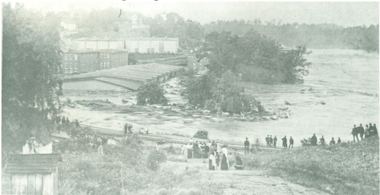
This scene taken with the photographer standing near where the present Rescue Squad building now stands. Hundreds of bales of cotton and cloth floated away with huge timber and machinery from Mills 1 and 2 during the flood of 1903. The bridge connecting both sides of the river went down also. The white painted stone cotton shed is the only building that stands today.
